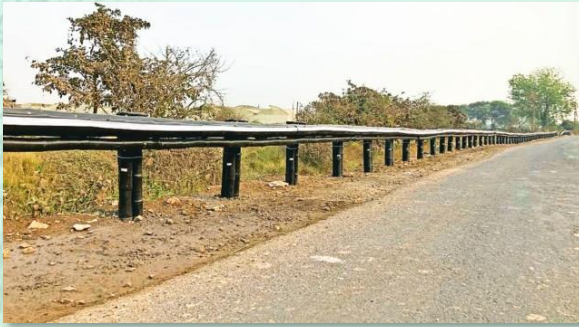
World's first bamboo crash barrier in India.
